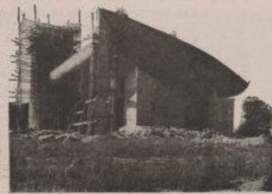
1. The chapel under construction and before rendering the walls, which are of load-bearing masonry taken from the old chapel. 2. Opposite, plan and axonometric superimposed as a view across the east wall, with the hotel towards Switzerland.
