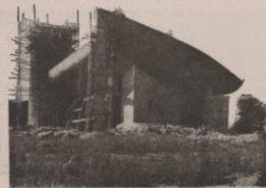
1. The chapel under construction and before rendering the walls, which are of buck-bracing stone taken from the old chapel. 2. Opposite, plan and axonometric superimposed as a view across the east wall, west the hotel towards Switzerland.
